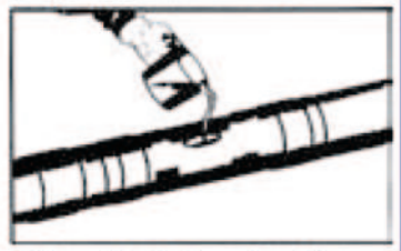
4) After waiting for the cooling of the sockets, pour the polyethylene (polyoleo-isocyanate) into the pipe, then the half of a cup of PE must be inserted into the gate and when the foam reaches the gate, push the whole plug.
